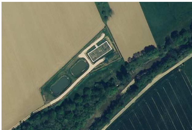
Station d'épuration de Baraton-Treigneux
