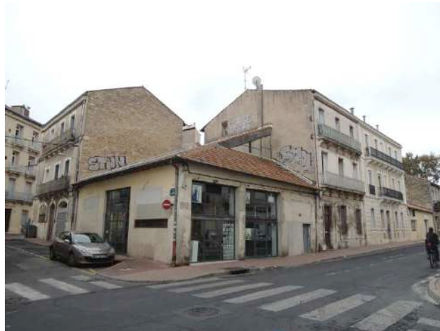
Restructuration de hangar
